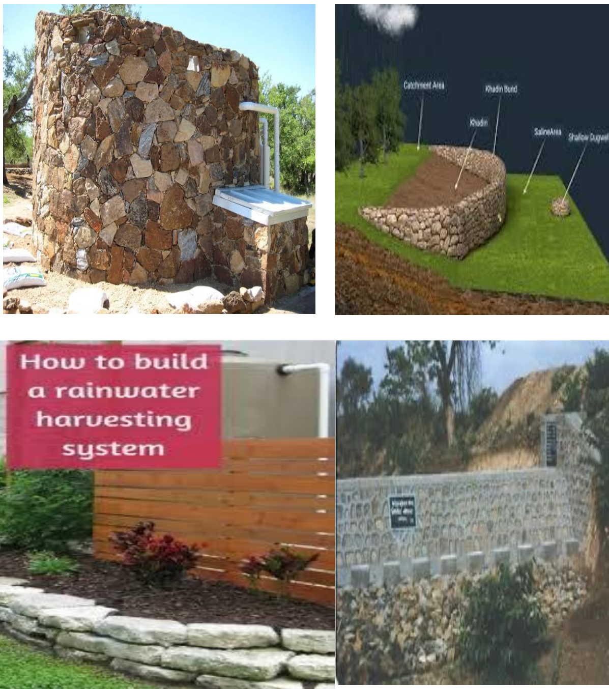
Picture 4: Using local stones (called magic stones in the area) for devising water harvesting systems
